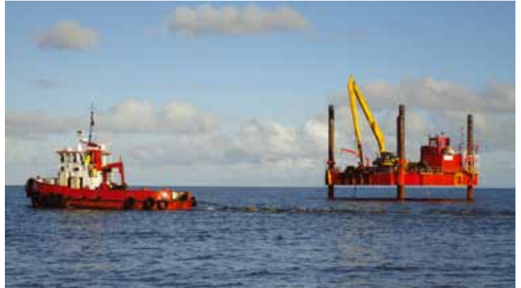
Pipeline being towed into position in preparation for installation on the seabed
